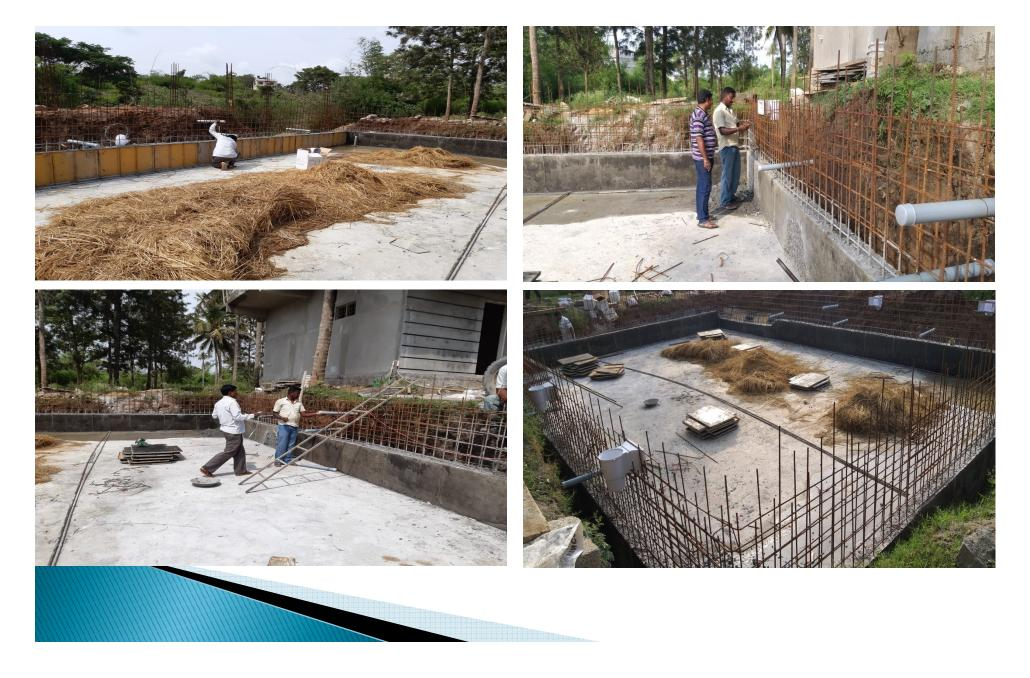
Fixing of pool fitting points including skimmer box, Centering frame fixing for 2<sup>nd</sup> level of wall concrete
