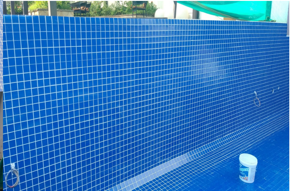
Pool View after Grouting.
