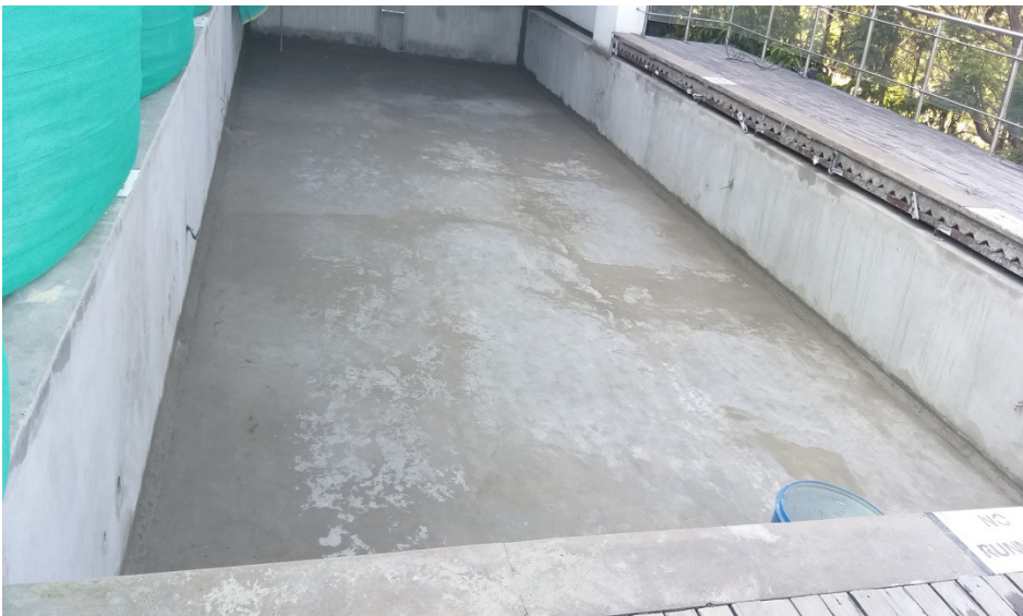
View of Plastering Completed pool
