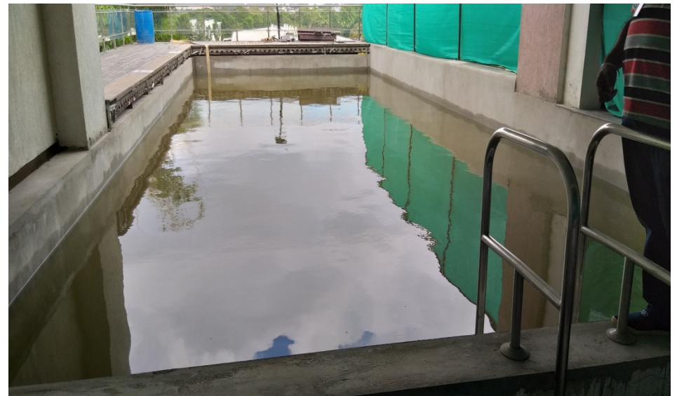
Water filled in pool for curing & Leakage checking
