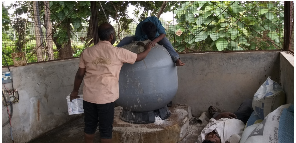
Electrical Control panel setup, removal of old media sand from filter
